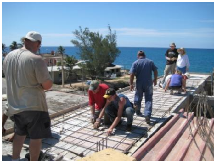
Tying rebar in preparation for concrete pouring.
